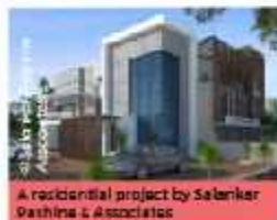
Use of fins and punched windows as fenestration on the western facade to create an optimal window to wall ratio
